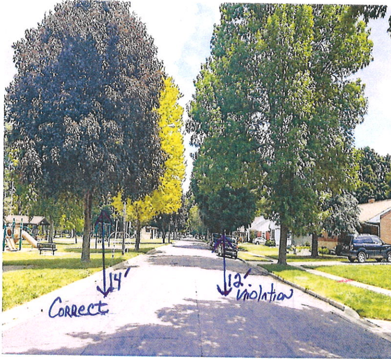
Height measurements for trees along township roads from Curb line up 14' Feet per Ordinance # 21-401
